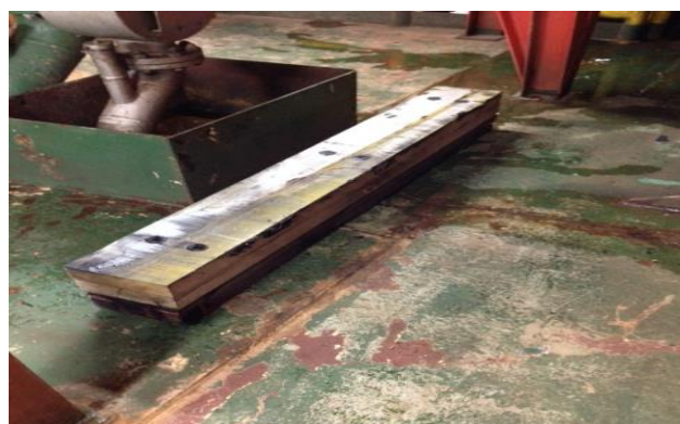
CRANE REST CHOCK WHICH FELL
