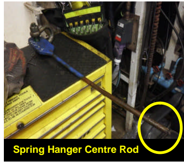
Position of failed Spring Hanger
