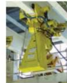
BOP chain hoist
