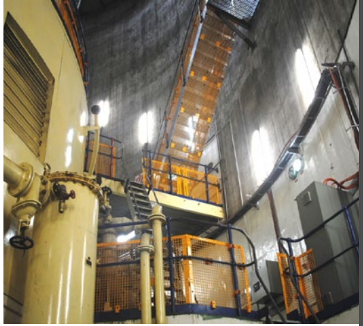
BLH Stop Drop™ Barricading installed on Stairways
