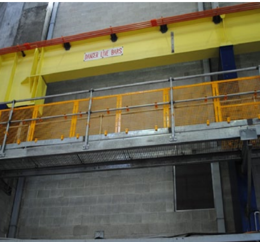
BLH Stop Drop™ Barricading installed on Walkways
