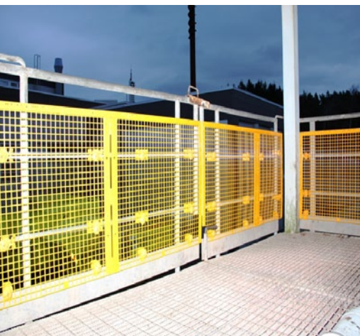
BLH Stop Drop™ Barricading installed on Platforms
