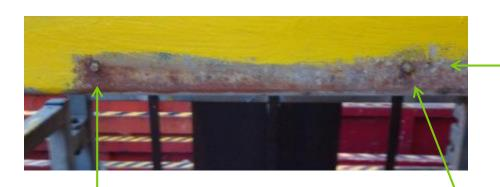
Due to corrosion on this bolt the rig team believe that this bolt was sheared prior to transit.
