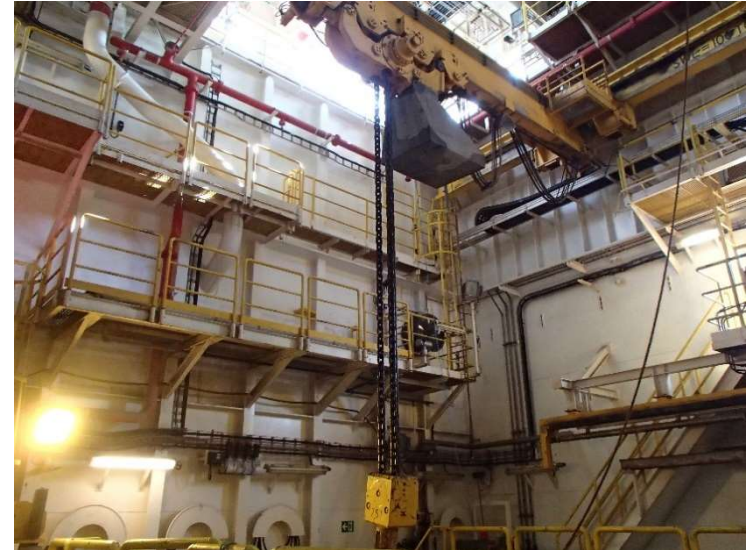
BOP Gantry Crane
