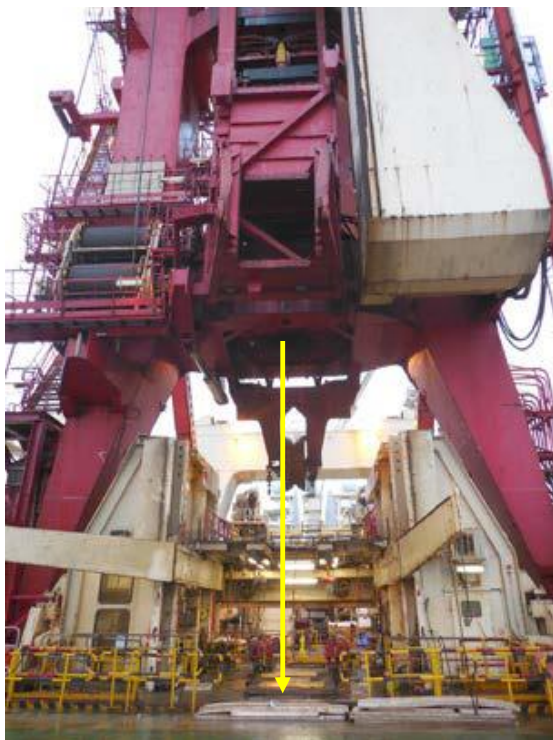
Figure: pipelay tower showing where hammer fell
