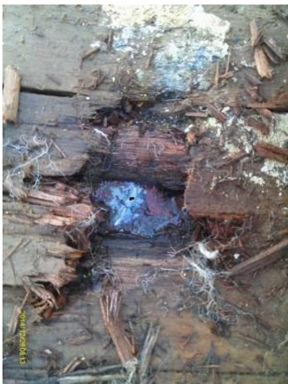
Figure: showing damage to deck
