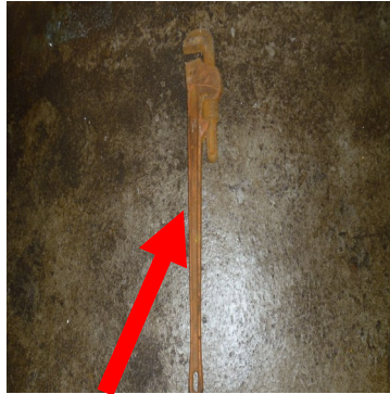
Stilsons that dropped from cable tray
