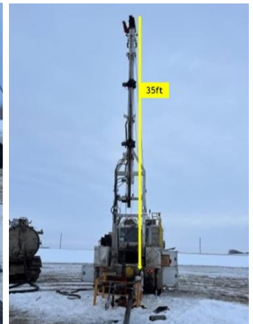
View of the lifting equipment mast
