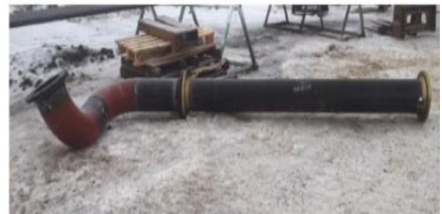
Example of pipe dropped off stands
