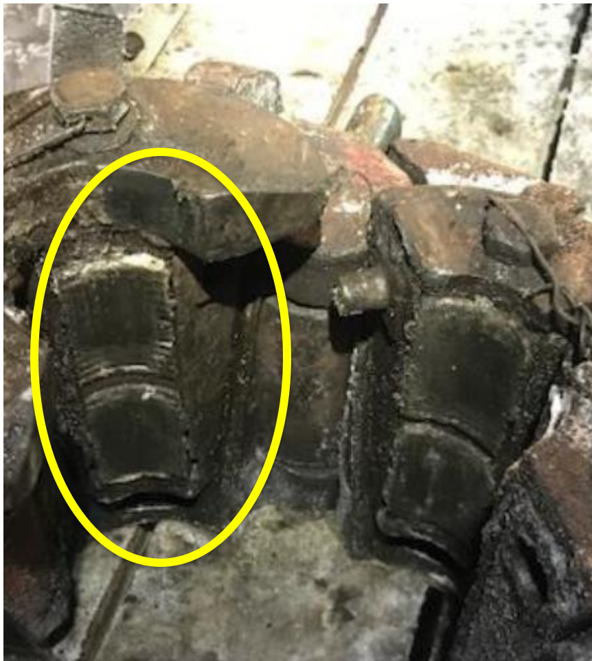
DAMAGED ELEVATORS, NOTICE INSIDE CONDITION OF ELEVATOR DIES
