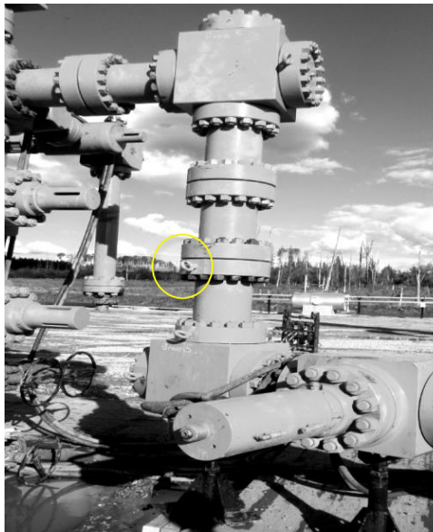
EYEBOLT LOCATED ON WELLHEAD
