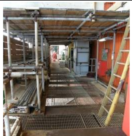
Worksite showing scaffold rack
